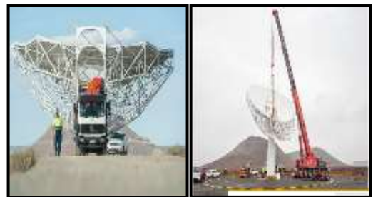
The first antenna (MeerKAT) for the Square Kilometre Array (SKA) project being wheeled out of the hangar, transported and erected by a massive crane in the Karoo desert.
